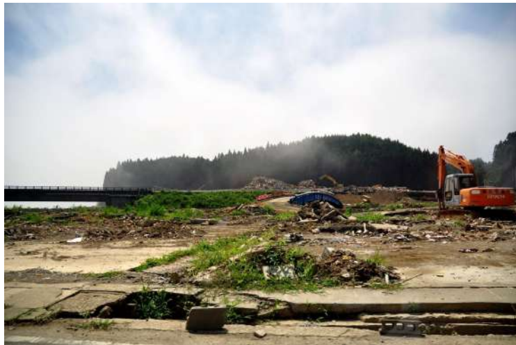
Reconstruction of widespread destruction in Tohoku
